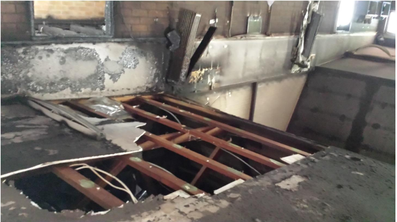
Burned roof damaging the roof
