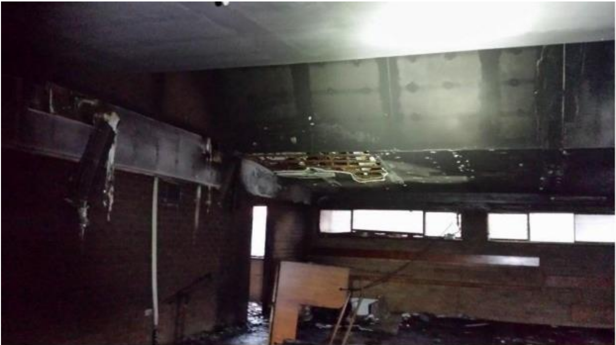
Burned ceiling and aircon machines
